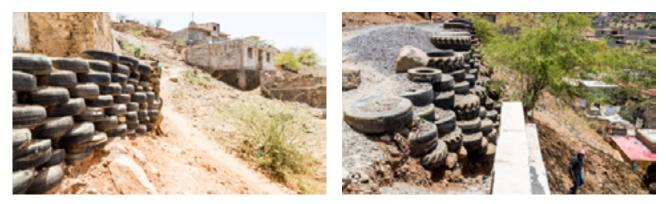
Picture 10: These improvised erosion mitigations might not withstand torrential rainfall. Houses below are directly at risk.
