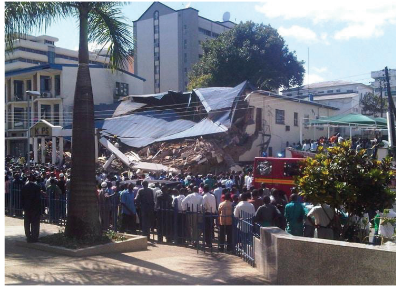
FIGURE 7: Collapsed Restaurant in Blantyre
