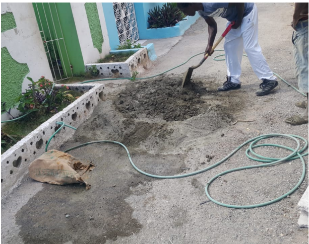
Photos 15 and 16: The photos above show the way concrete is most frequently mixed. Dosage is usually by rule of thumb, but the ratio of cement is generally fair. Mixing is irregular at best. Dry concrete is often reincorporated into the mix. Mixes are usually too wet.
