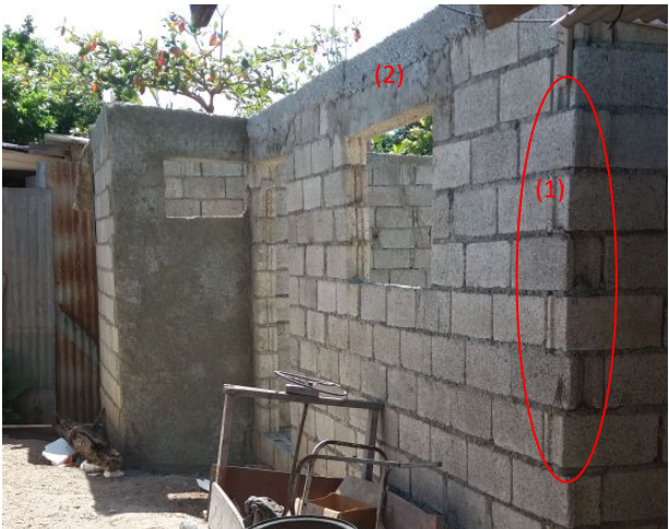
Photo 7: It's common to find unconfined corners (1) in many houses. Masonry is generally reinforced with vertical steel bars every other block cell, but these are usually not properly filled, negating many if not all of the benefits. It's also common to see a window lintel directly under the ring beam (known as "belt" beam in Jamaica). They can be poured separately or together. The addition of the lintel in this case may not bring great benefit. The steel and concrete could perhaps have been used in more important locations.
